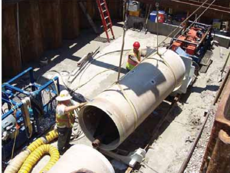
2 Figure 6-7. Typical Jack and Bore Casing Installation
