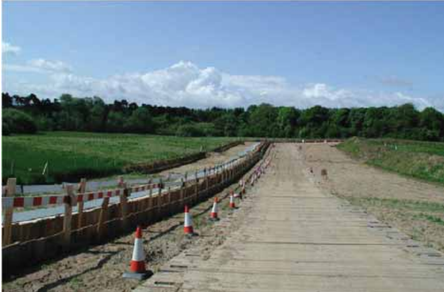
1 2 Figure 6-4. Typical Cable Construction ROW with Single Cable Trench Open
